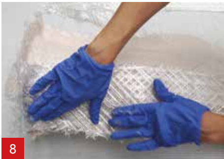
8 ...and apply a 2nd layer of A1 Triaxial fibre on the still wet A1.
