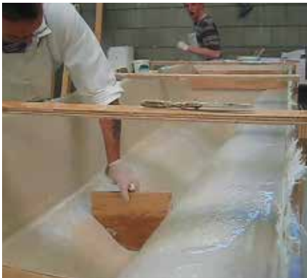
Construction inside panel Mahler - The Netherlands
